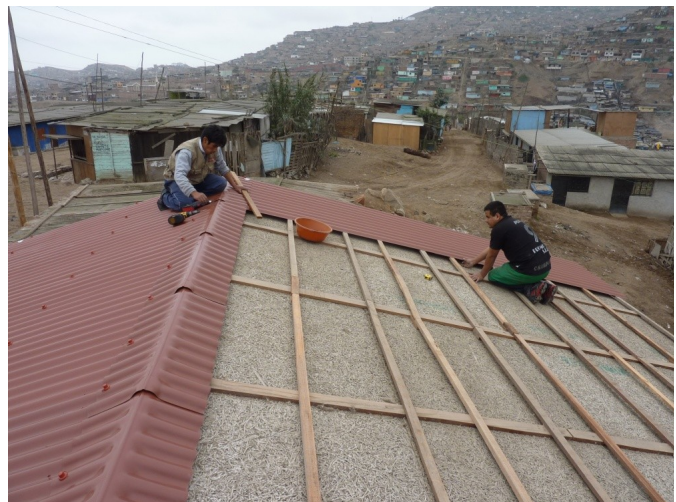
Hooligan resistant polycarbonate plates
